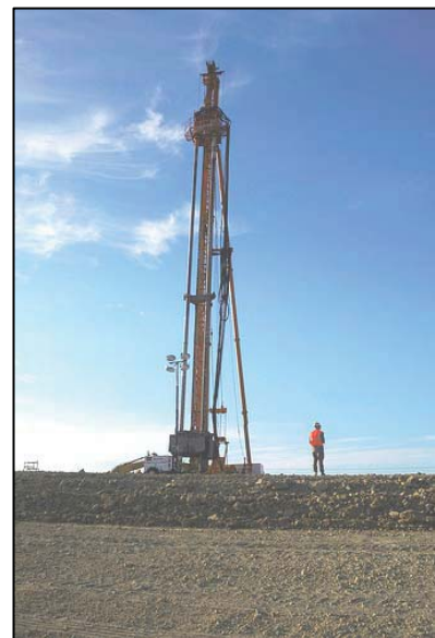
Photograph 4-3. Deep soil mixing equipment
